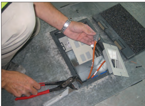
Full EMC protection to the floor outlet.
